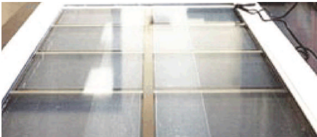
Removed Sections of Preserve at Grille Locations
